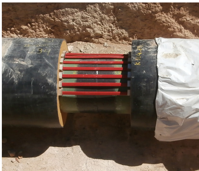
Figure 6. Cables transiting pipe joint.
