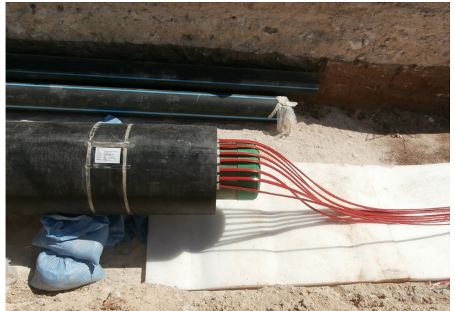
Figure 5. Cable feed point.
