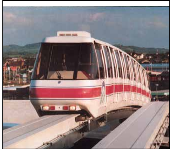
Heated Monorail Track Using Heat Trace's Longline Series Resistance, Constant Power Output Heater
