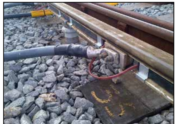
120CRH7 Self-regulating Contact Rail Heater Installed on 3rd Rail for London Underground
