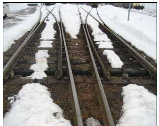
Typical Points Heating System in Operation
