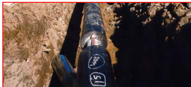
Buried, Pre-insulated Pipe with Longline HTS3F
