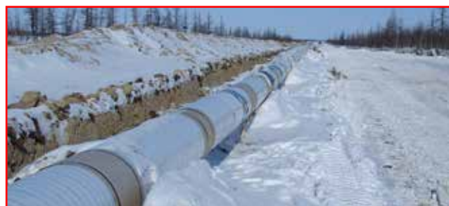
Completed Skin Trace system prior to burying
