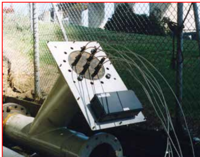
Internal pipe tracing
