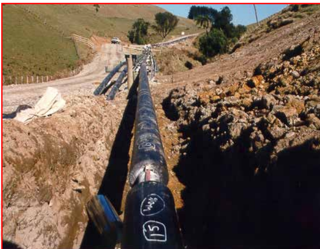
Buried pipeline tracing
