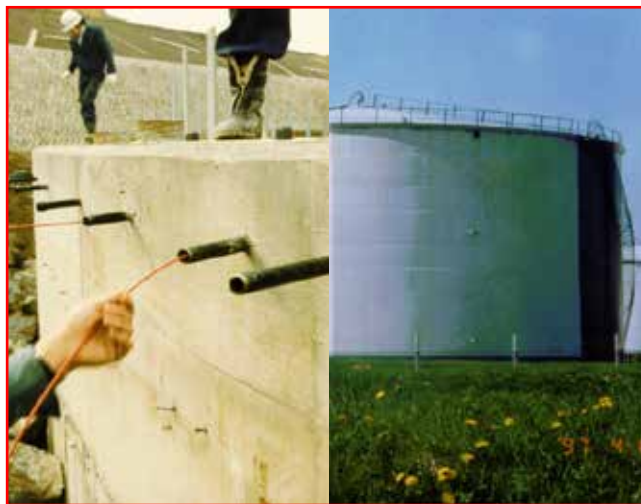
Tank base heating
