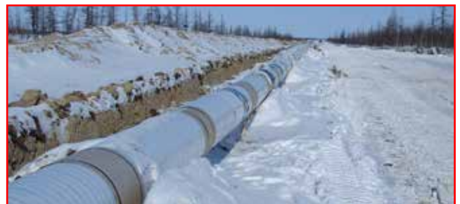
Completed Skin Trace system prior to burying
