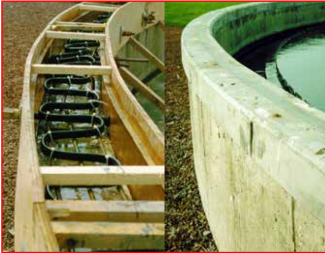
Final Settlement Tank de-icing
