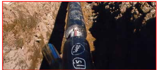
Buried, Pre-insulated Pipe with Longline HTS3F
