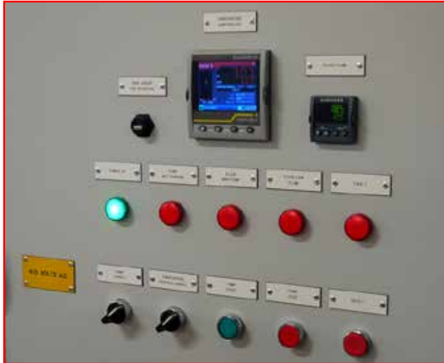
Control Panel for 3m Pipe Test Rig
