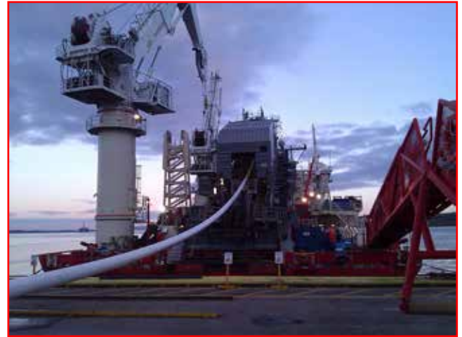
Completed electrically heat-traced pipe-in-pipe being reeled onto the pipelay vessel.
