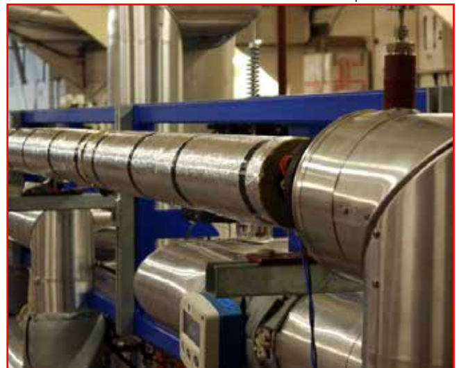
3m Pipe Test Rig
